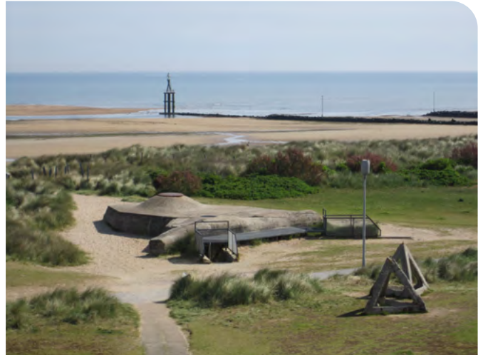
Observation bunker built in 1944. Photo taken in 2018.
